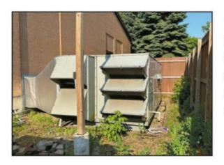
The HVAC system in the church was installed when it was built in 1997. The furnace and a/c unit servicing the west side of the church has failed and is obsolete. We must replace the west unit entirely to keep our congregation comfy year-round.
