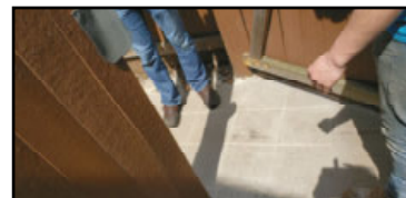
Gate reversed and pavers installed to facilitate opening when snow impedes access.
